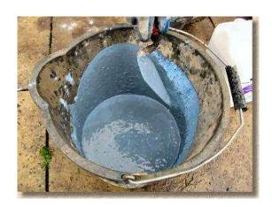
Mortar/screed: Mix cement and sand first, then add 'GIC SBR Extra' diluted with water refer to the mixing ratio table). Mix either by hand or with low speed drill for 2 to 5 mins.
