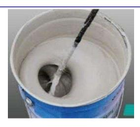
**Spatterdash:** Mix cement and sand first, then add 'GIC SBR Extra' diluted with water refer to the mixing ratio table). Mix either by hand or with low speed drill for 2 to 5 mins.
