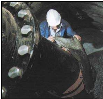
P1* application: Mastic Blanket on flange...
