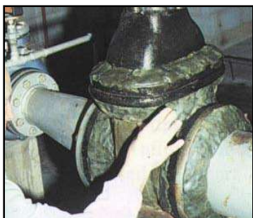
Profiling with Densyl Mastic.
