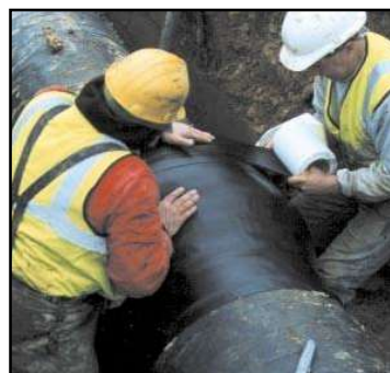
being overwrapped with Densoclad Tape...
