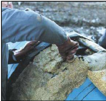
P1* application: Profiling Mastic on Tybar...
