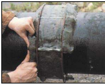
Profiling and infilling with Densyl Mastic.
