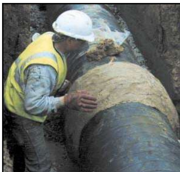
P2* application: Profiling Mastic on flange...
