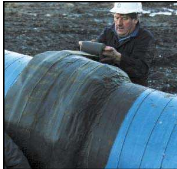
being overwrapped with Denso Tape...
