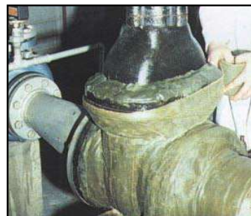
Overwrapping with Denso Tape
