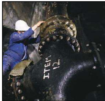
being overwrapped with Denso Tape...
