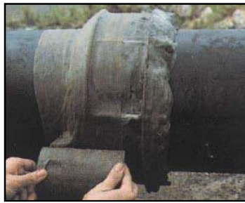
Overwrapping with Denso Tape
